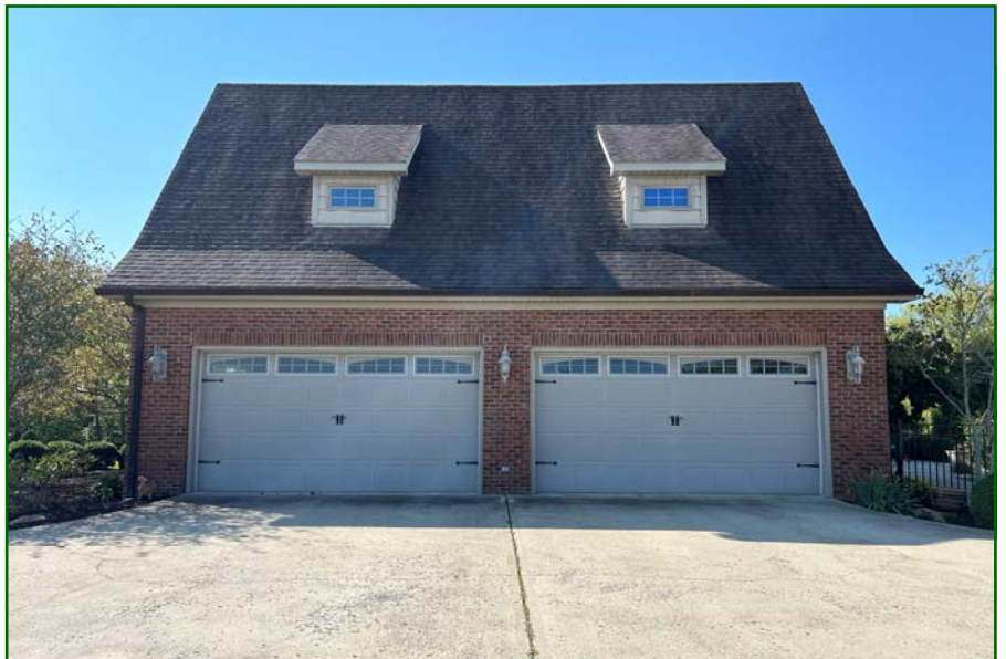
Four-car attached garage with concrete floor, window blinds, wire shelving
